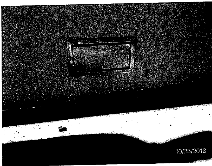
TYPICAL FLOOD VENT
